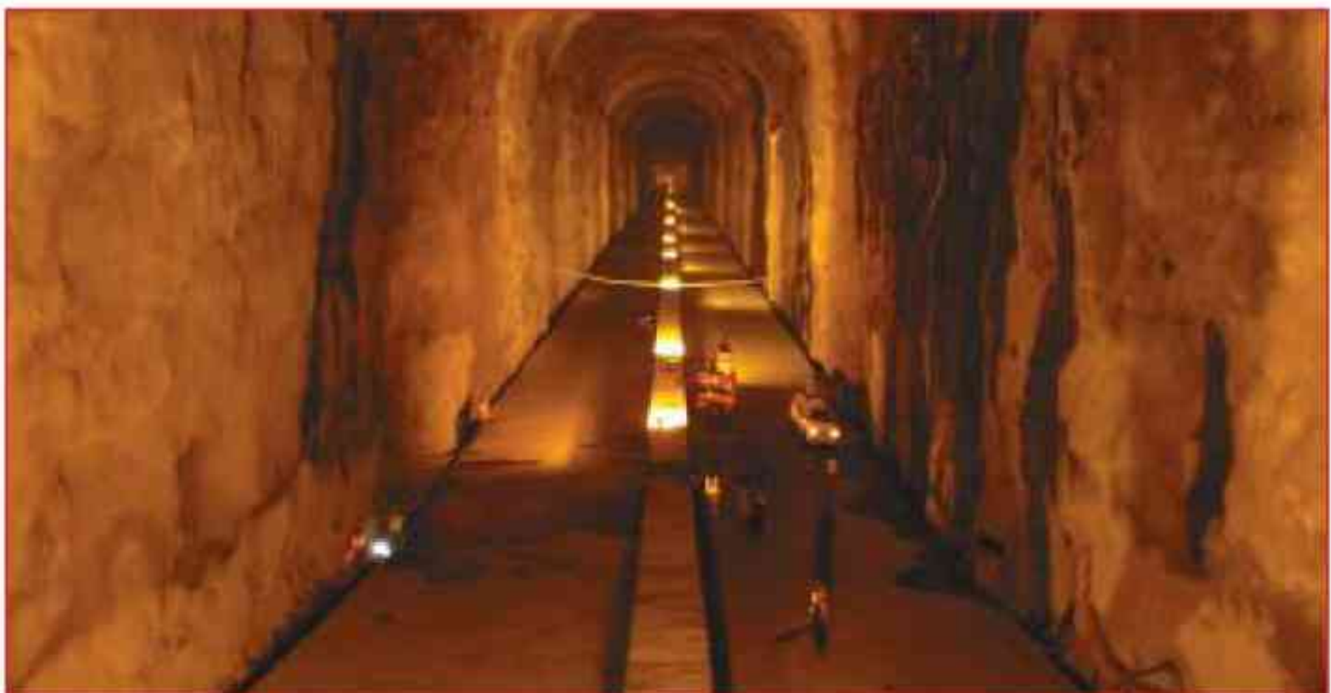
Underground Crude oil storage Rock Cavern view of Padur
